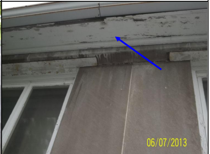
Photo 4 – Soffit with deterioration. This board should be replaced with the roofing project.
